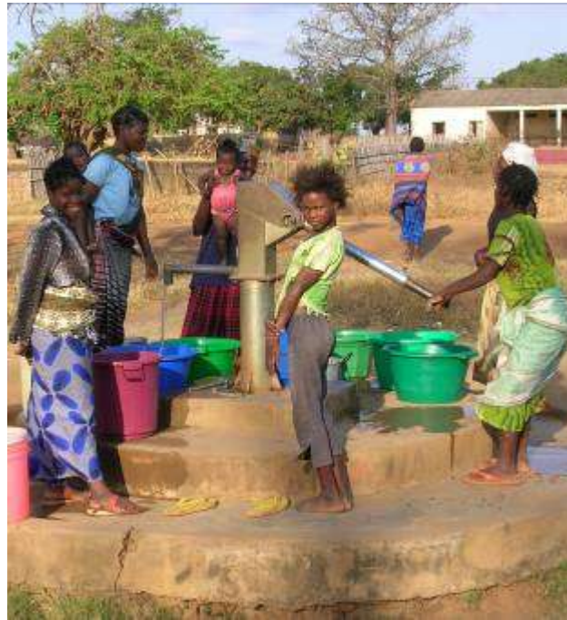
Afridev Pump (Mozambique)
