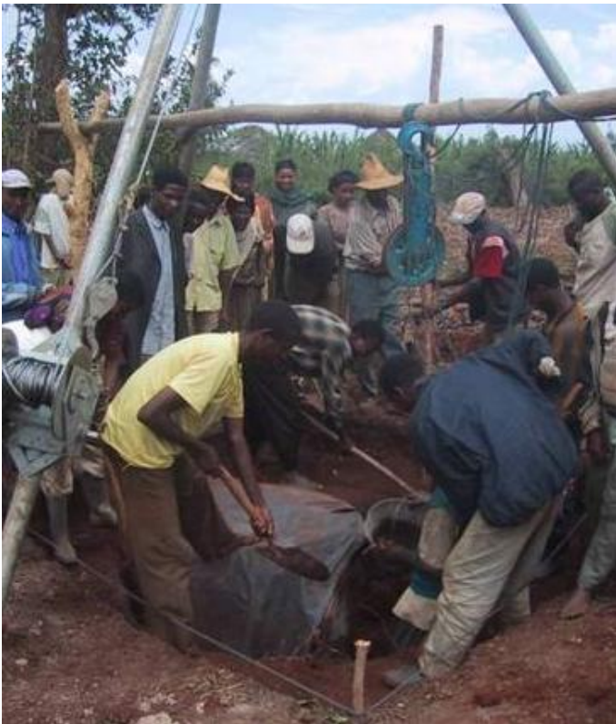
Figure 2: Community Constructs a Hand Dug Well
