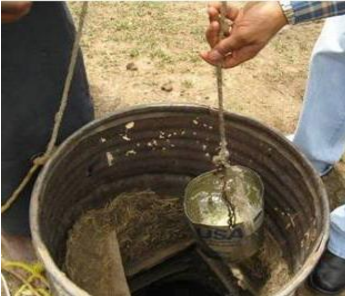
Figure 3: Traditional Well - Protected and Stabilised
