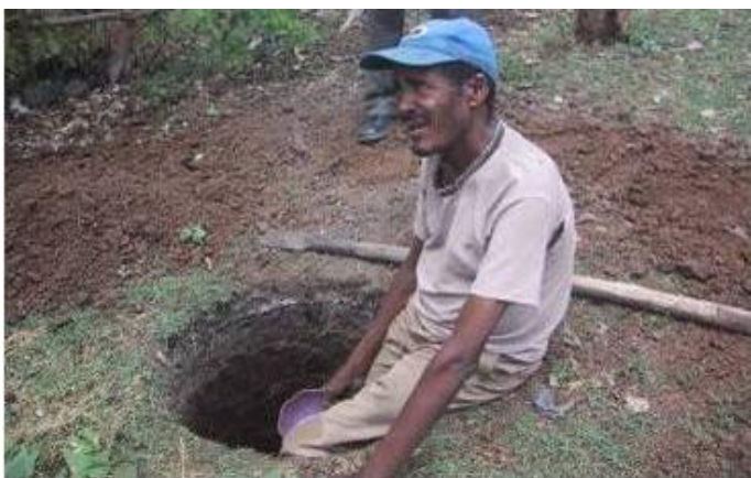
Figure 4: Small Diameter Well-Digging in Ilu Woreda
