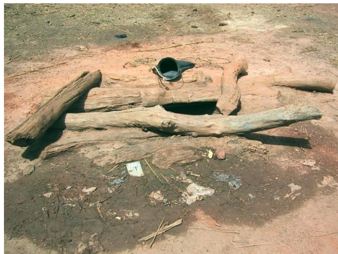
Figure 3: A typical unlined traditional hand dug well
