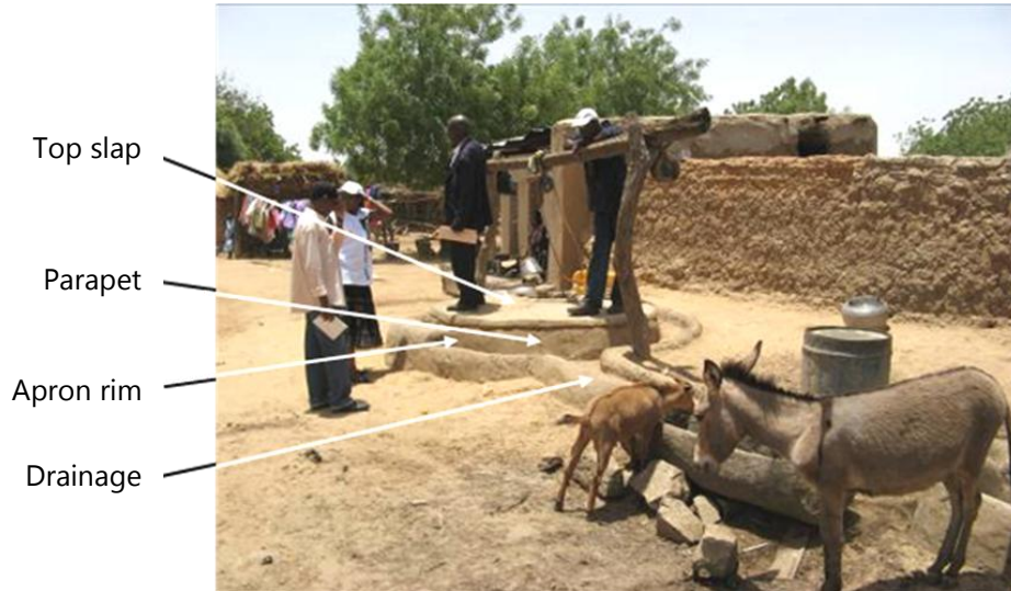
Figure 5: Example of an up-graded well in Mali
