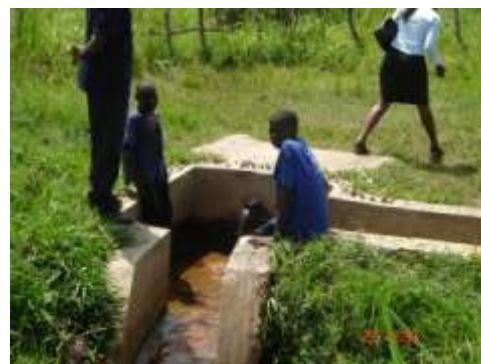
A community spring in Amuria district. Community contributed land, sand, stones, labour, delivery pipe and fencing
