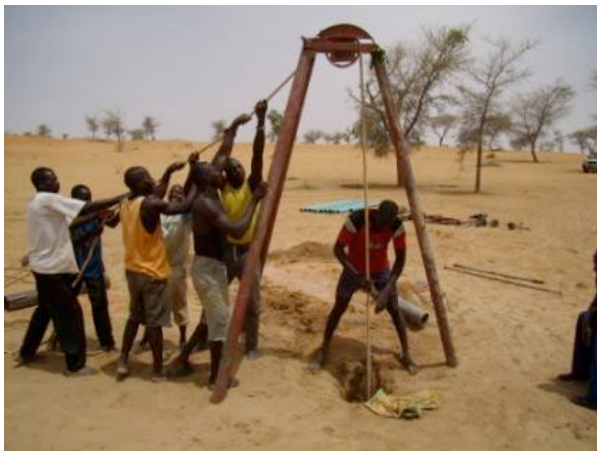
Hand Percussion Drilling in Lalawa, Niger (Photo: Enterprise Works/VITA)
