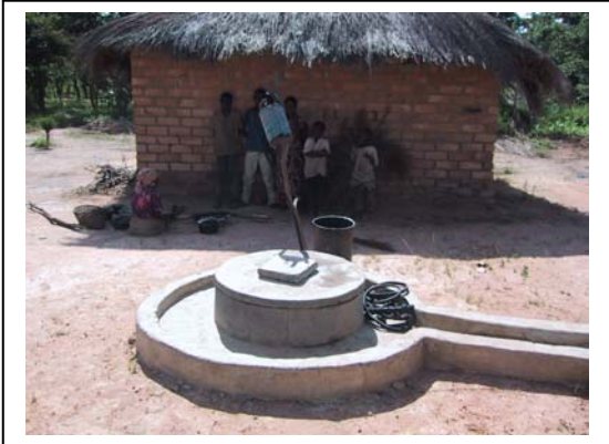
Simplest level of source improvement. Near to house for all uses. costs less than $250
